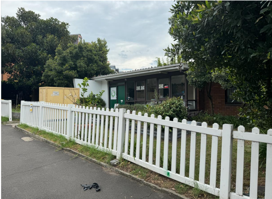
Figure 2: Site viewed from Lower Fort Street
